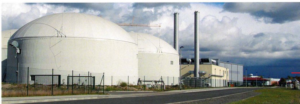
APG and bio-gas power plant
